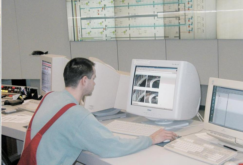
In the control center at the Kaiserslautern central sewage plant, the live images are compared to stored images of the target situation.
